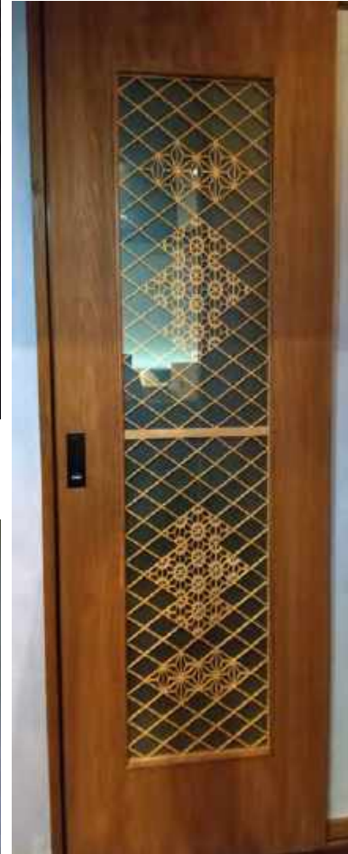
Wooden Muntin On Sliding Door Window
